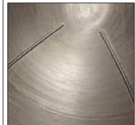
3/4" rods welded in place
